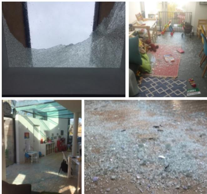
Figure 1. Examples of shattered rooflights
